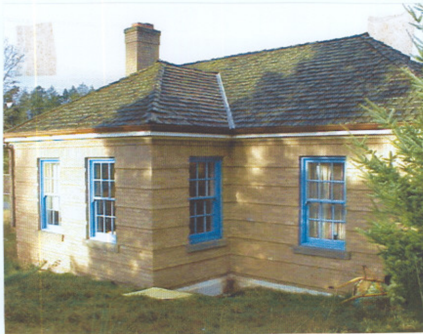
2 Building 38, Colwood; rear view ( CFB Esquimalt, March 2000. )
