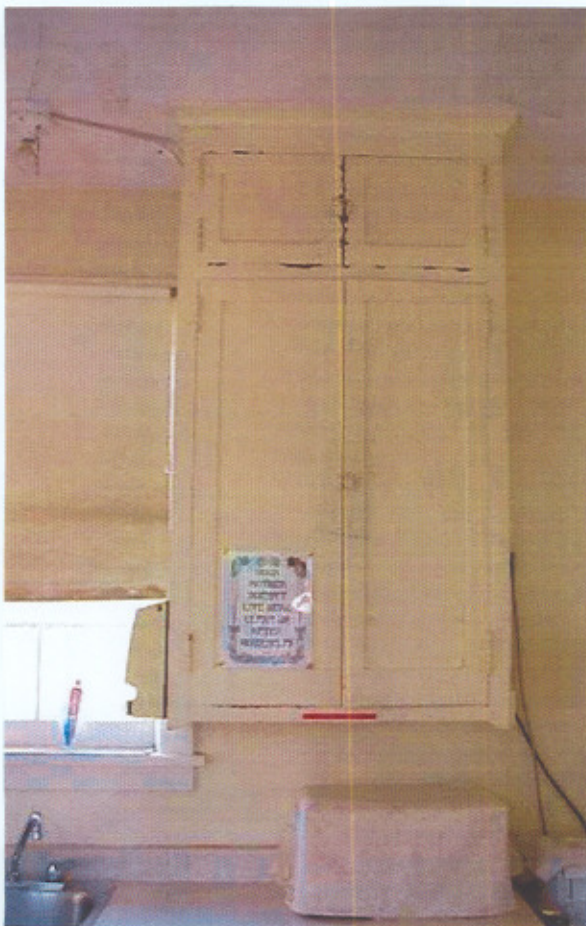
3 Building 38, Colwood; kitchen cupboard. ( CFB Esquimalt, March 2000 )
