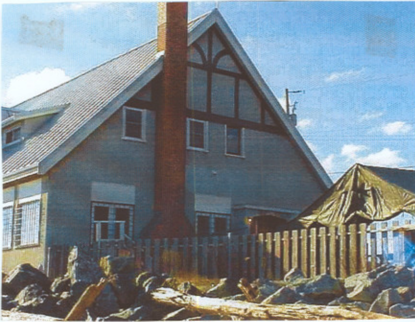
8 Building 602, south and east sides (CFB Esquimalt, Feb. 2000)
